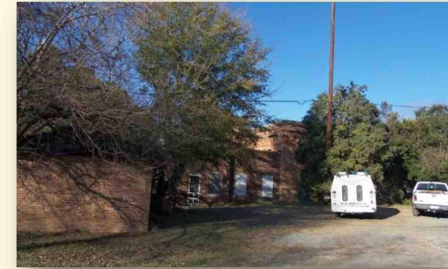
Steam Plant – Before (2013)
