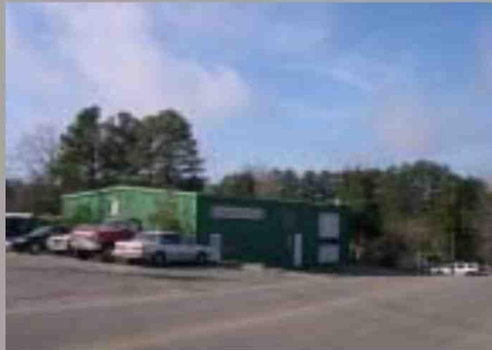
Former rescue squad facility
