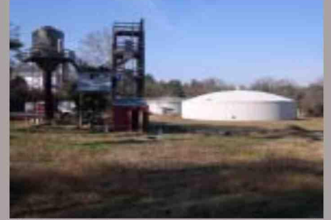
Firefighting training tower & county water tank
