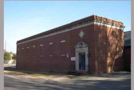
Sprint telecommunications facility
