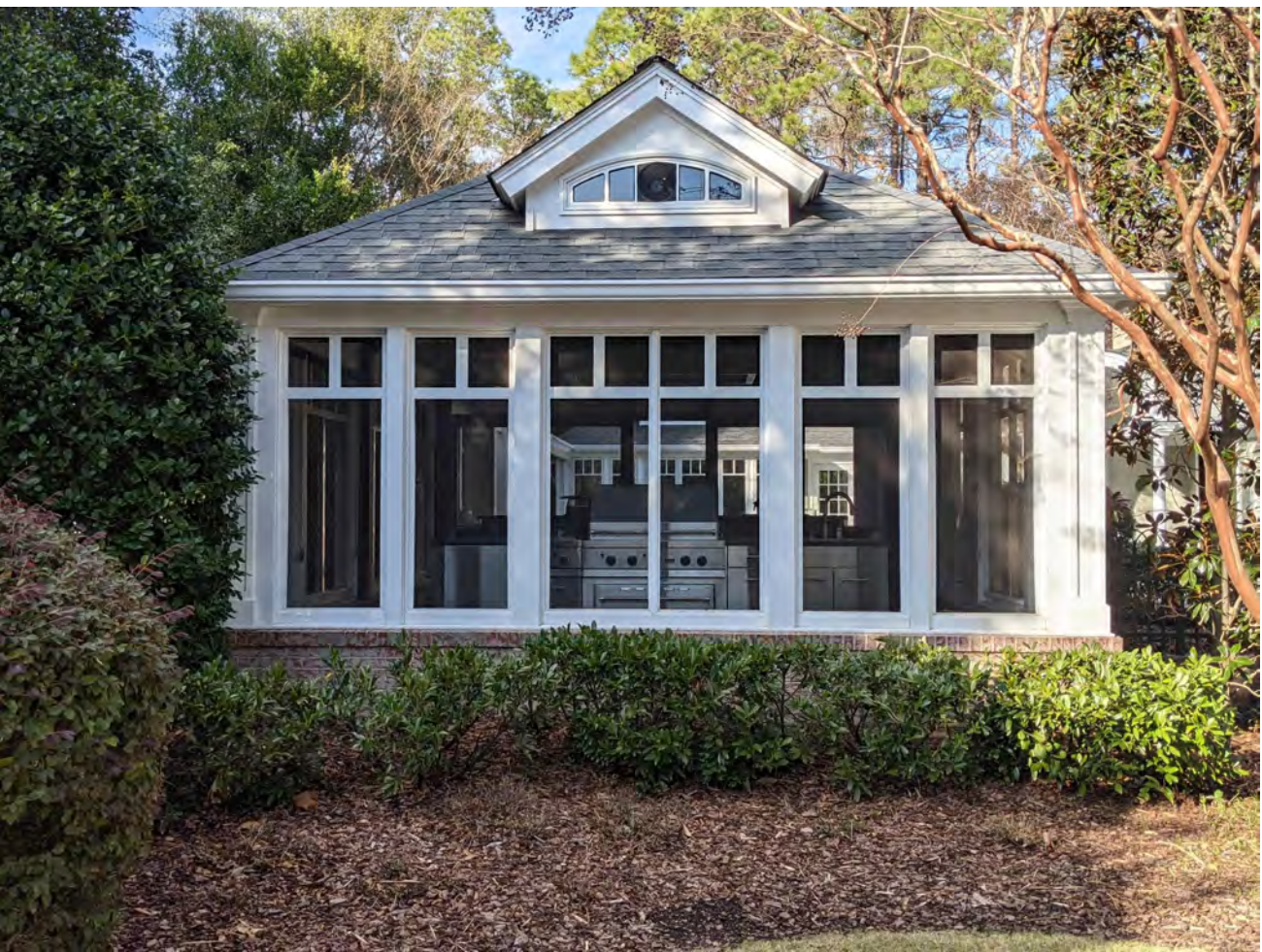
2. EXAMPLE OF SCREEN PORCH WALL SYSTEM
