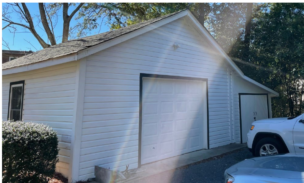
Existing garage door on outbuilding (Exhibit A-3.6)
