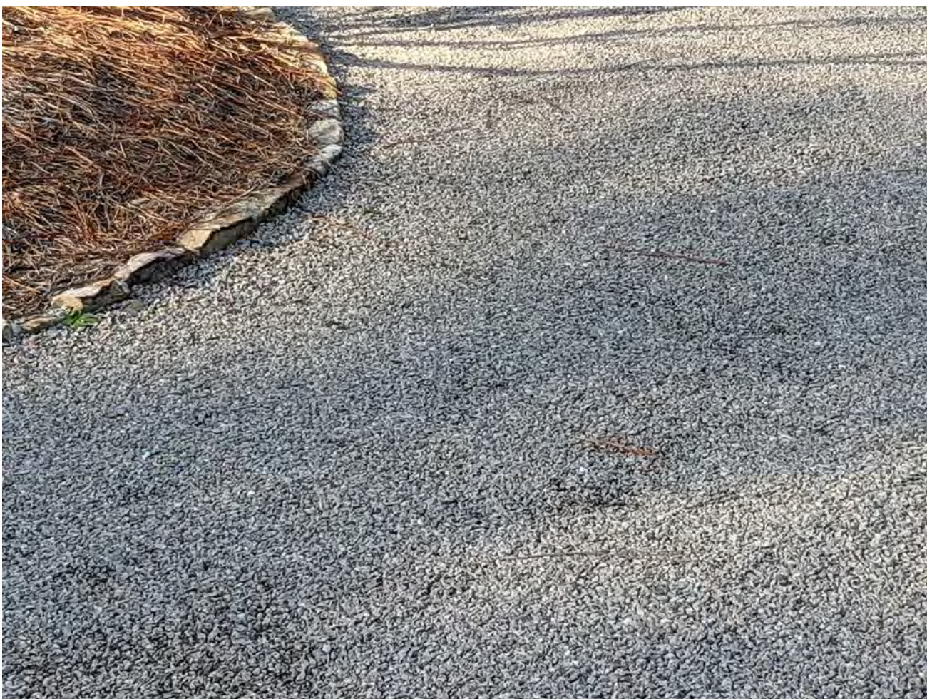
11. DRIVEWAY GRAVEL & CURB
