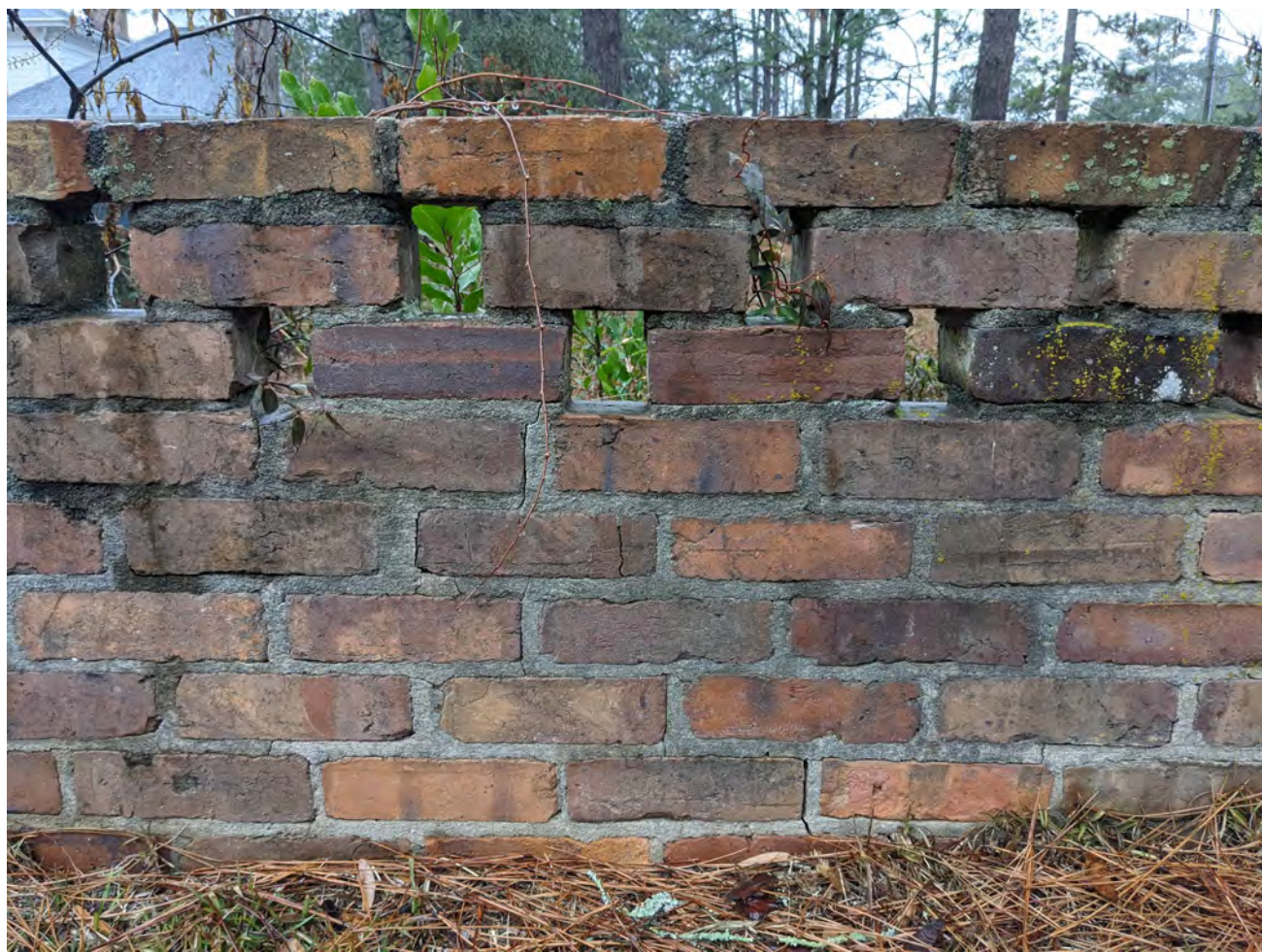
1. BRICK PERIMETER WALL & LATTICE
