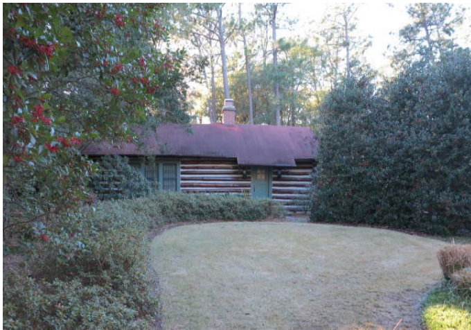
FRONT VIEW OF THE EXISTING LOG CABIN.
