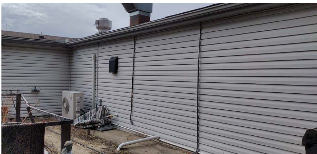
Rear of the building
