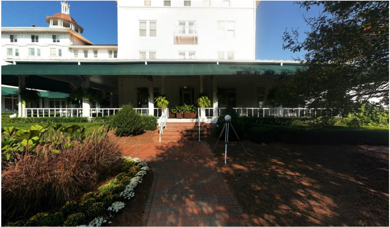
Existing (exterior view 3)
