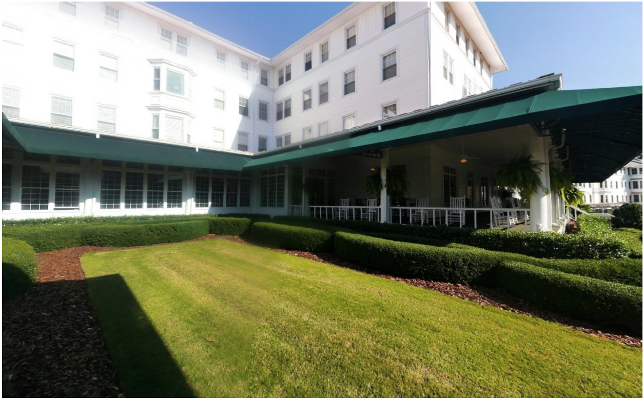
Existing (exterior view 2)
