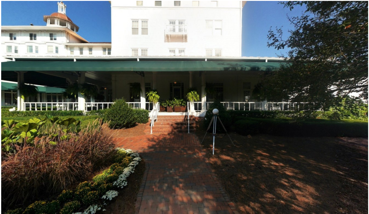
Existing (exterior view 3)
