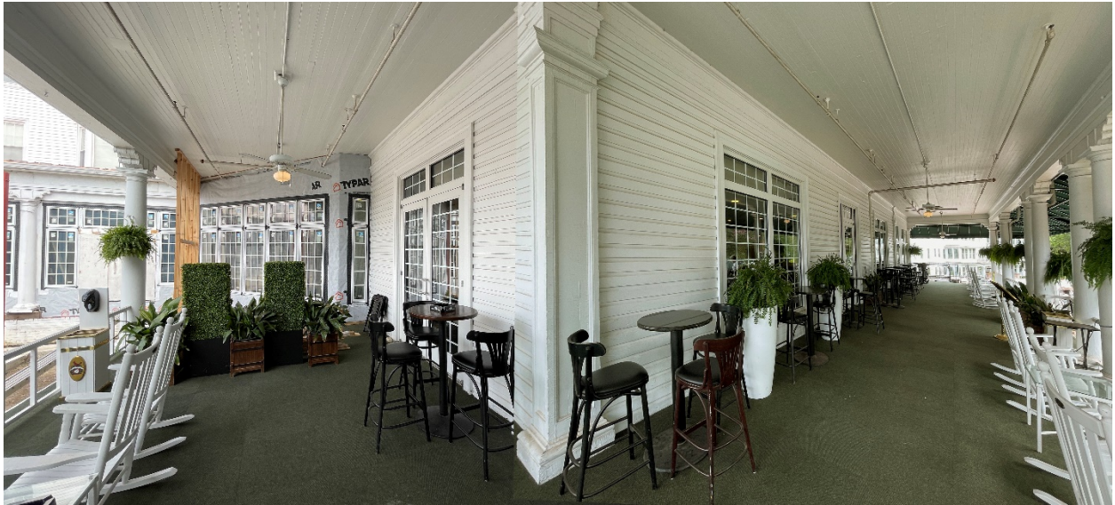
Existing (exterior view 1)
