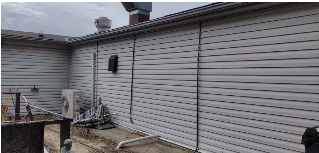
Rear of the building
