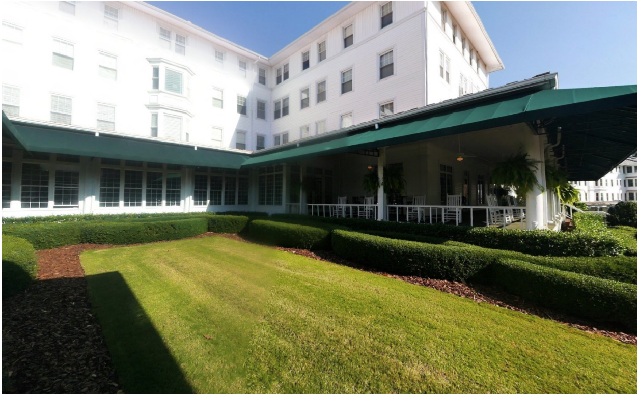
Existing (exterior view 2)
