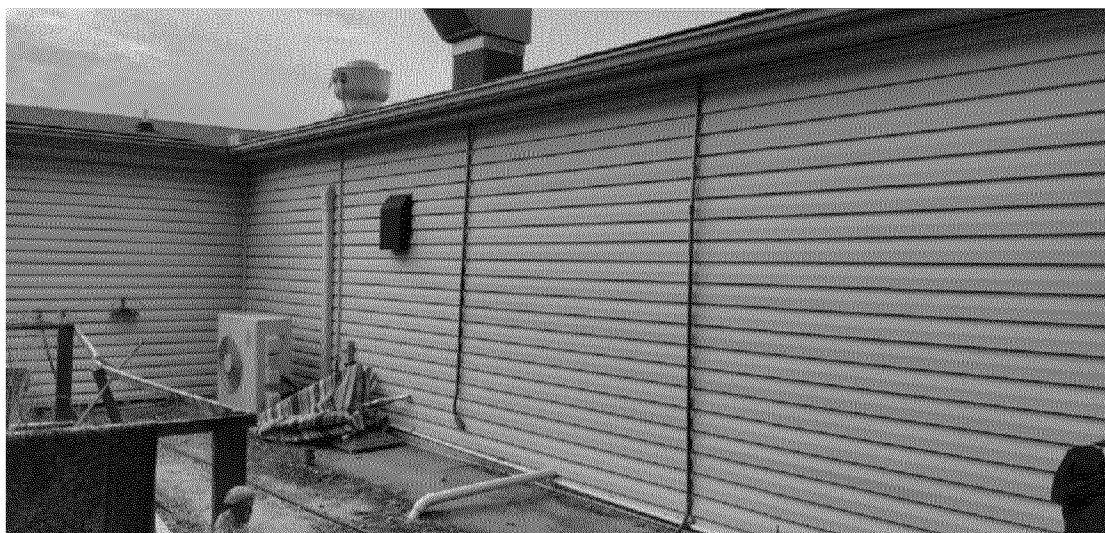
Rear of the building
