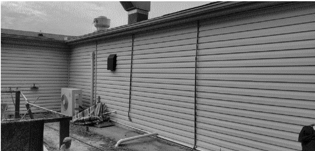
Rear of the building
