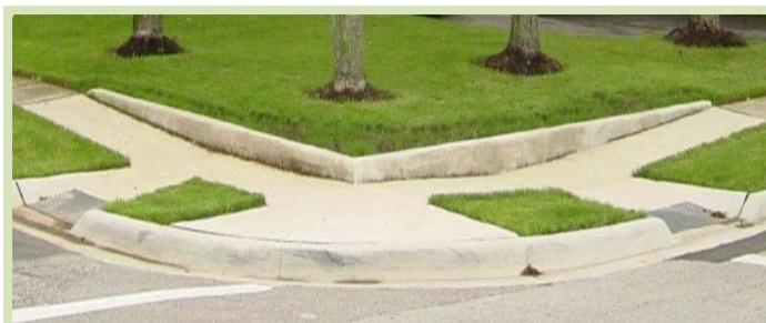
Properly constructed sidewalks are essential to Village connectivity.
