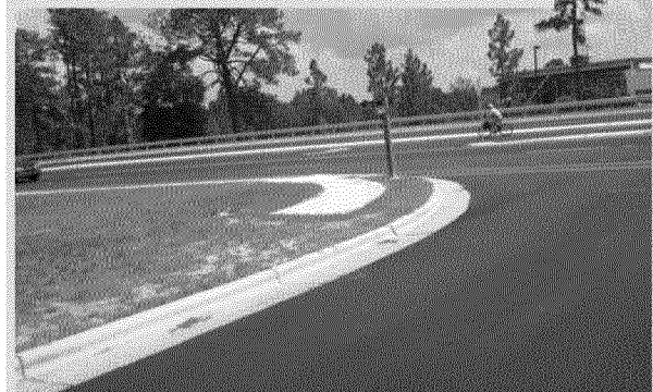
Recently completed sidewalk on NC 211 offers opportunity for connectivity.
