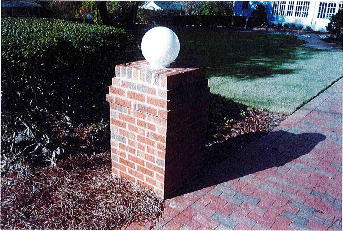
EXISTING ENTRY COLUMNS
