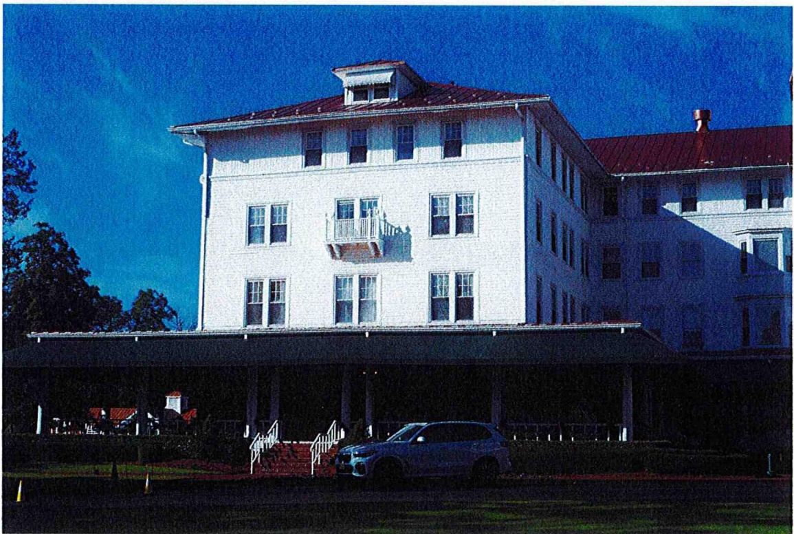
CAROLINA HOTEL: EXISTING JULIET BALCONIES
