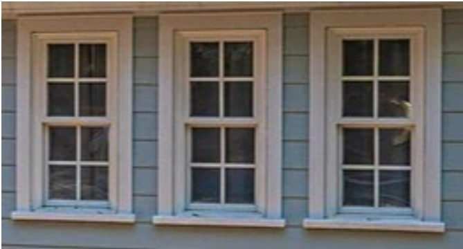
Double hung windows; with 4" trim on three (3) sides and sill board at the bottom
