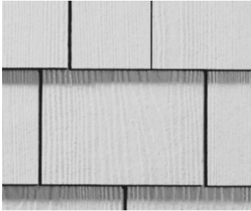
Front Elevation Siding Hardi-Board Shake
