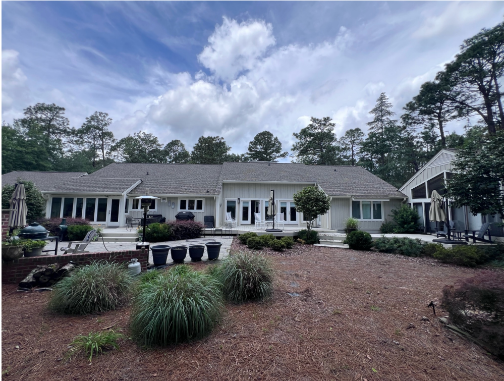
Current View of the back of the home
