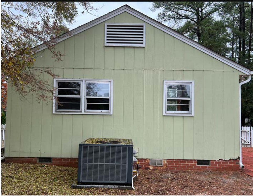
Picture of the rear of the property:
