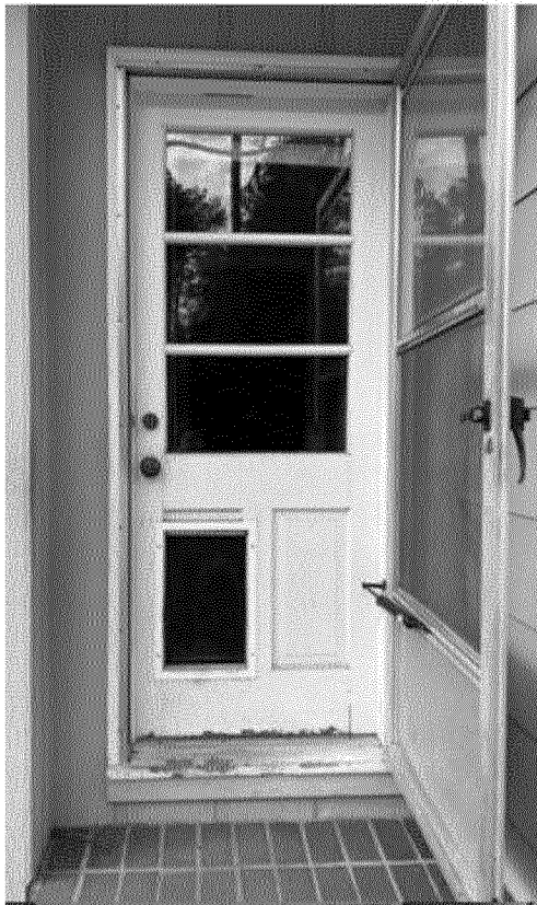
Picture of the current door to the side of the property:
