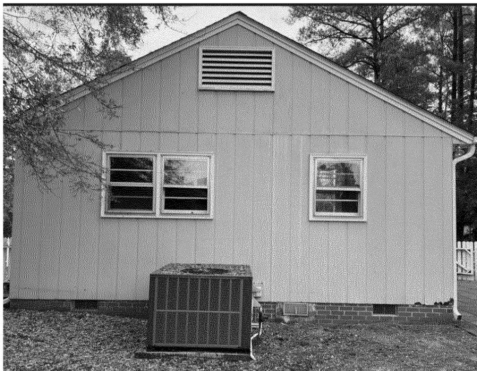
Picture of the rear of the property:
