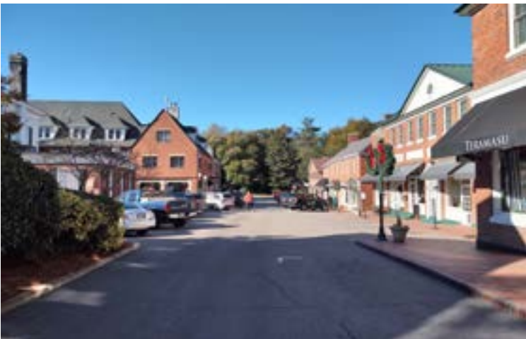
MARKET SQUARE TYPICAL SECTION (B) The widest part of Market Square has diagonal parking on each side of the one-way drive aisle. The brick sidewalk on the north side provides access to the shop. On the south side, the brick sidewalk provides access to alley cut-through to Chinquapin Rd. The sidewalks are narrow on both sides of the asphalt.
