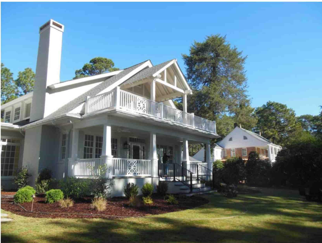
Rear porch and balcony addition
