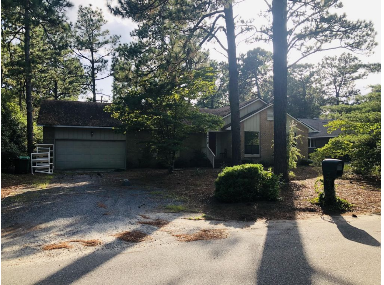
Existing home before renovation showing windows.
