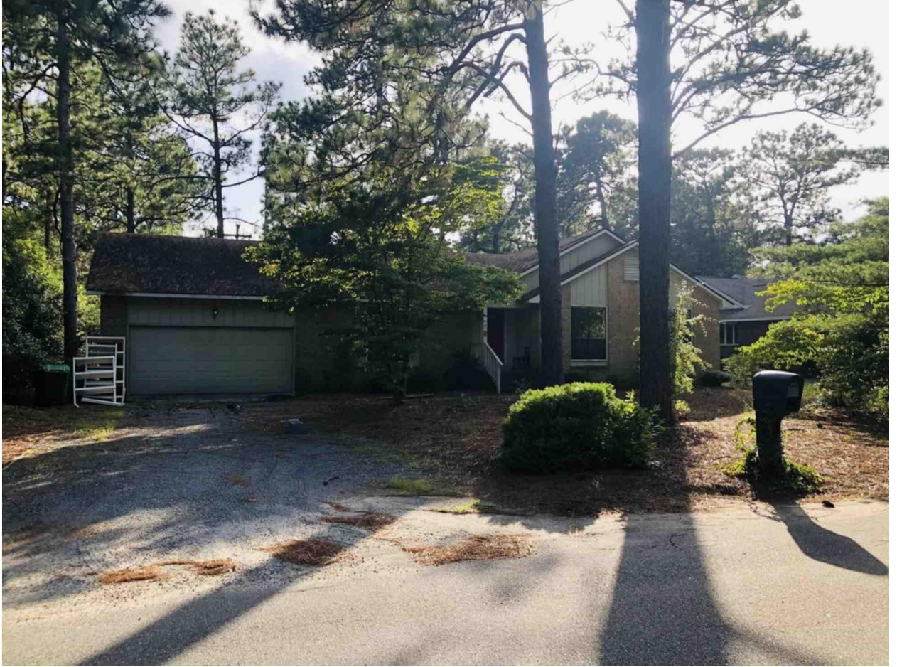
Existing home before renovation showing windows.
