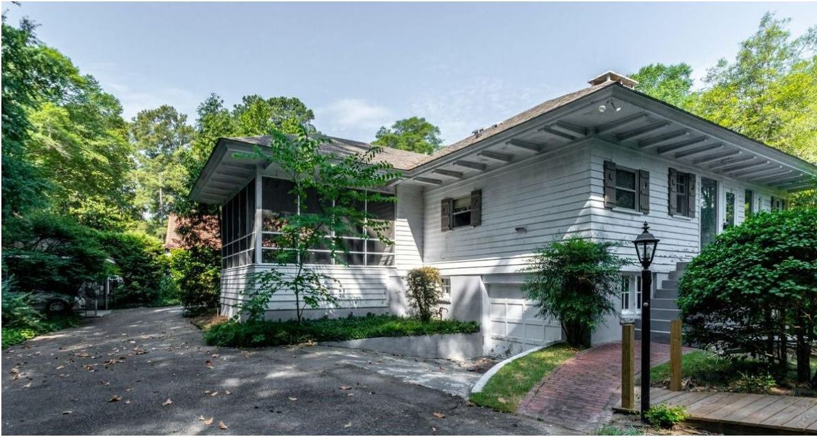
Existing Left Side & Left Rear
