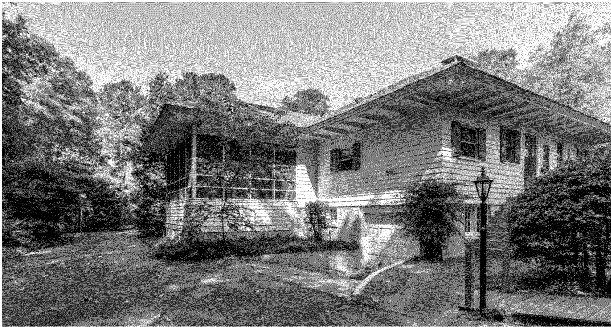
Existing Left Side & Left Rear
