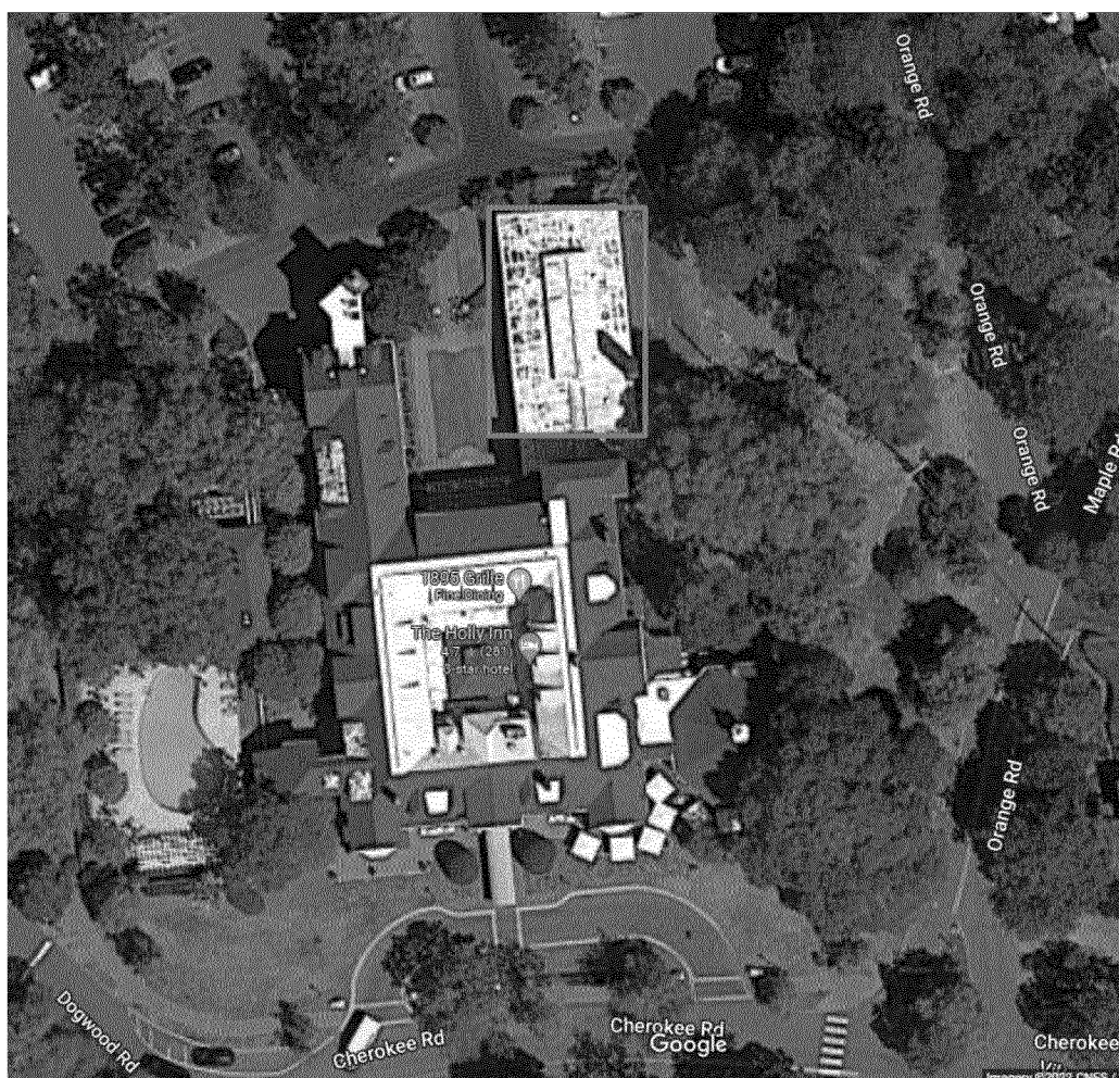
Aerial view of the proposed hotel roof replacement
