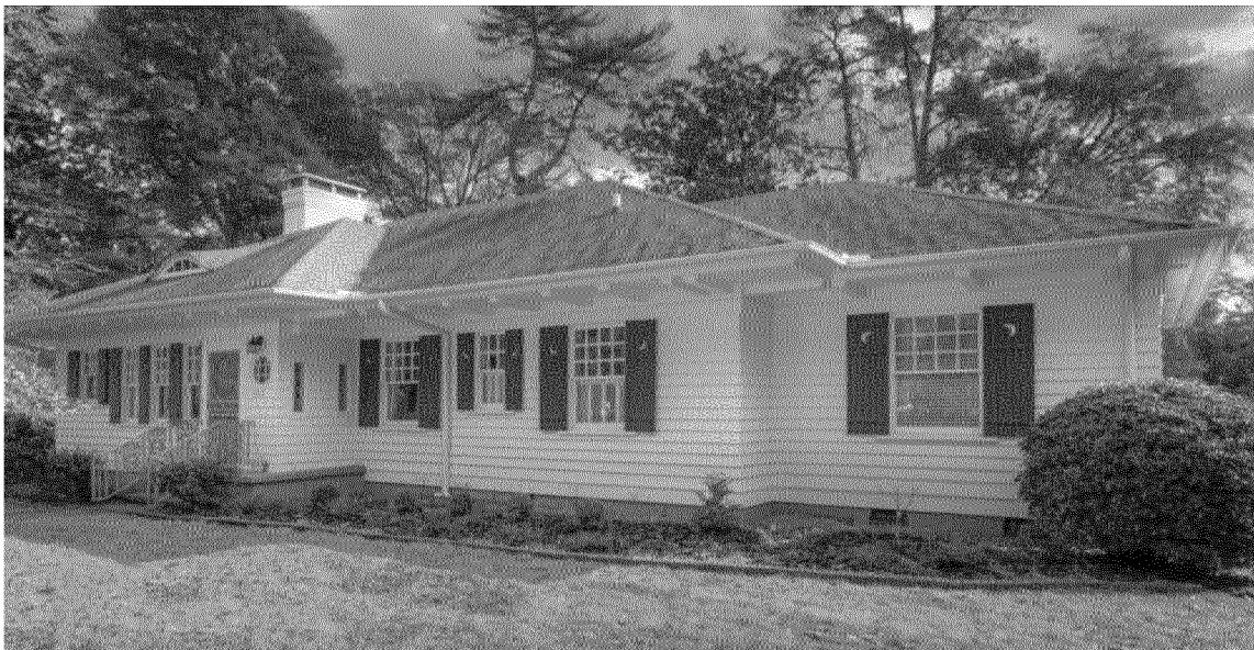
Existing Front of House
