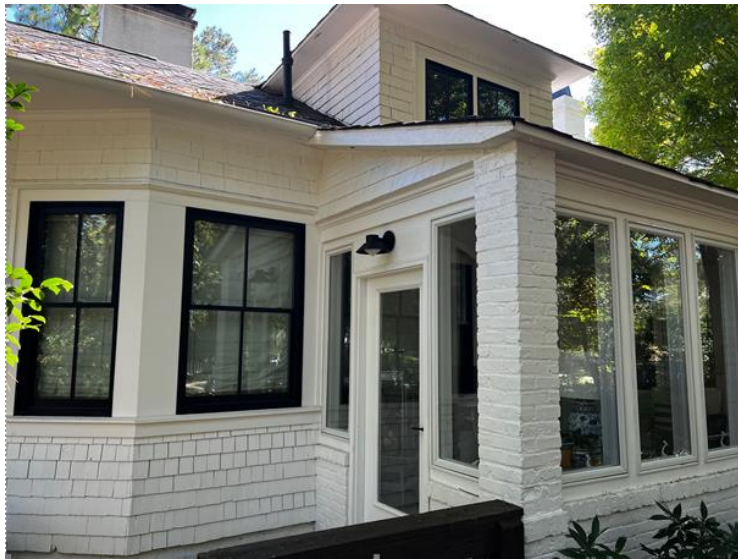
Picture J: Picture of the side of the the main structure:
