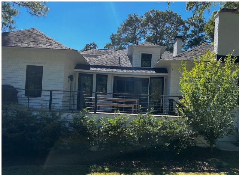
Picture I: Picture of the rear of the the main structure:
