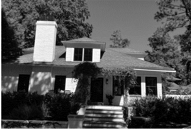
Picture H: Picture of the front of the the main structure:
